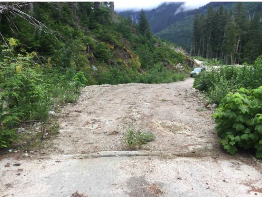
Left Approach Facing Away From Bridge
