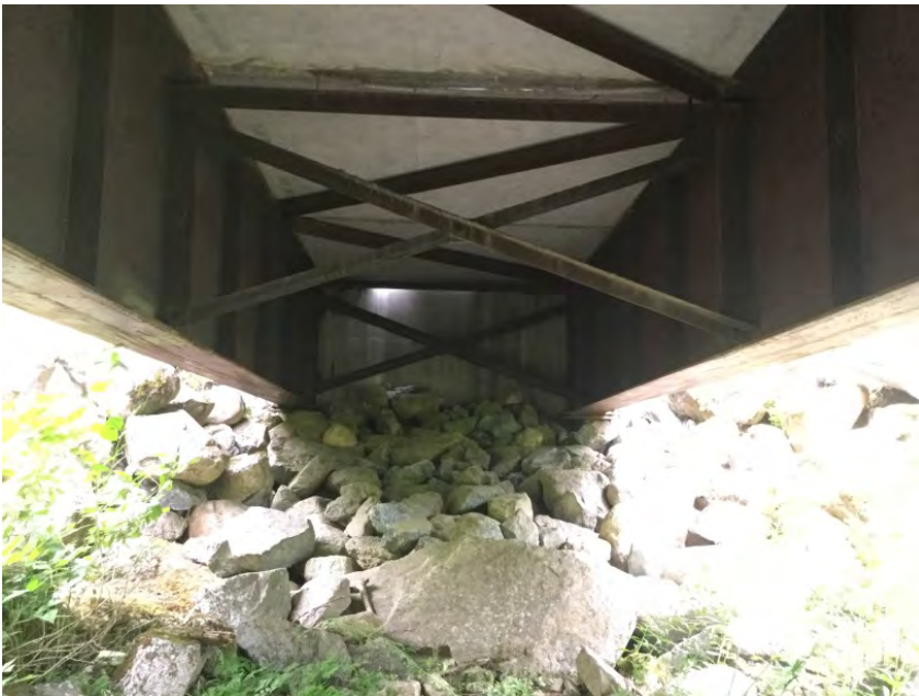
Left Bank Abutment
