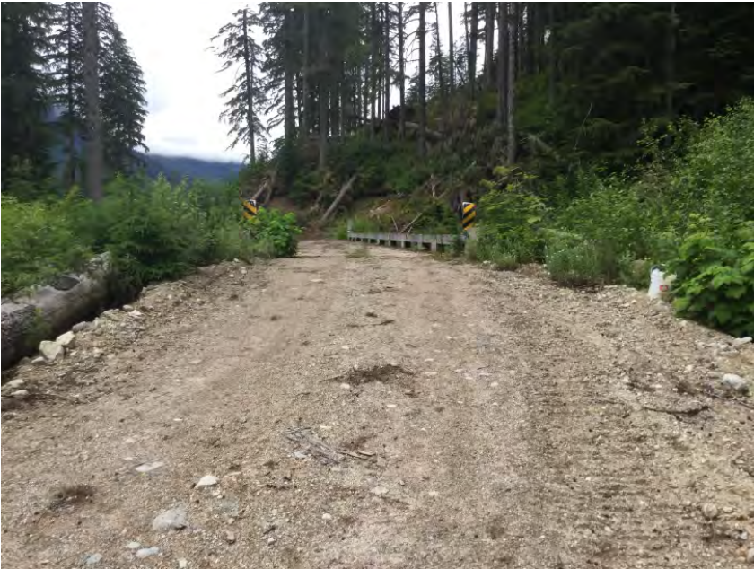
Left Approach Facing Bridge
