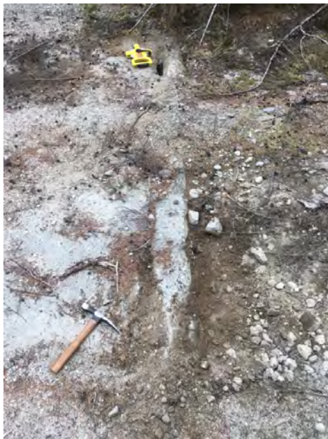
Damage to Right Abutment Ballast Wall & Deck Panel
