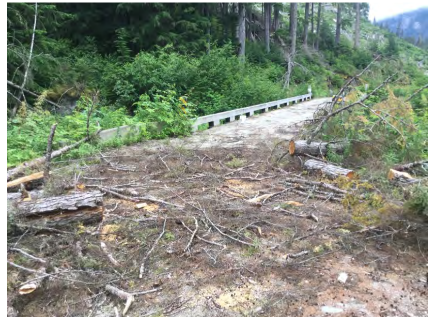
Right Approach Facing Bridge
