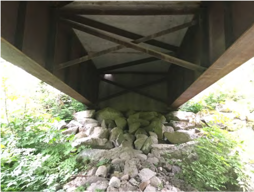
Right Bank Abutment
