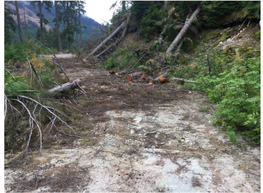
Right Approach Facing Away From Bridge
